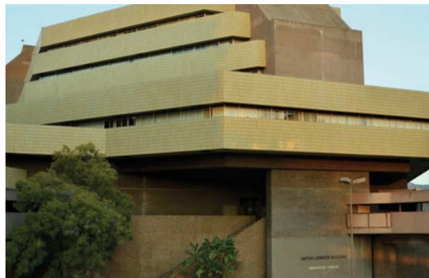
Anton Lembede Building, Muckleneuk Campus, Tshwane
