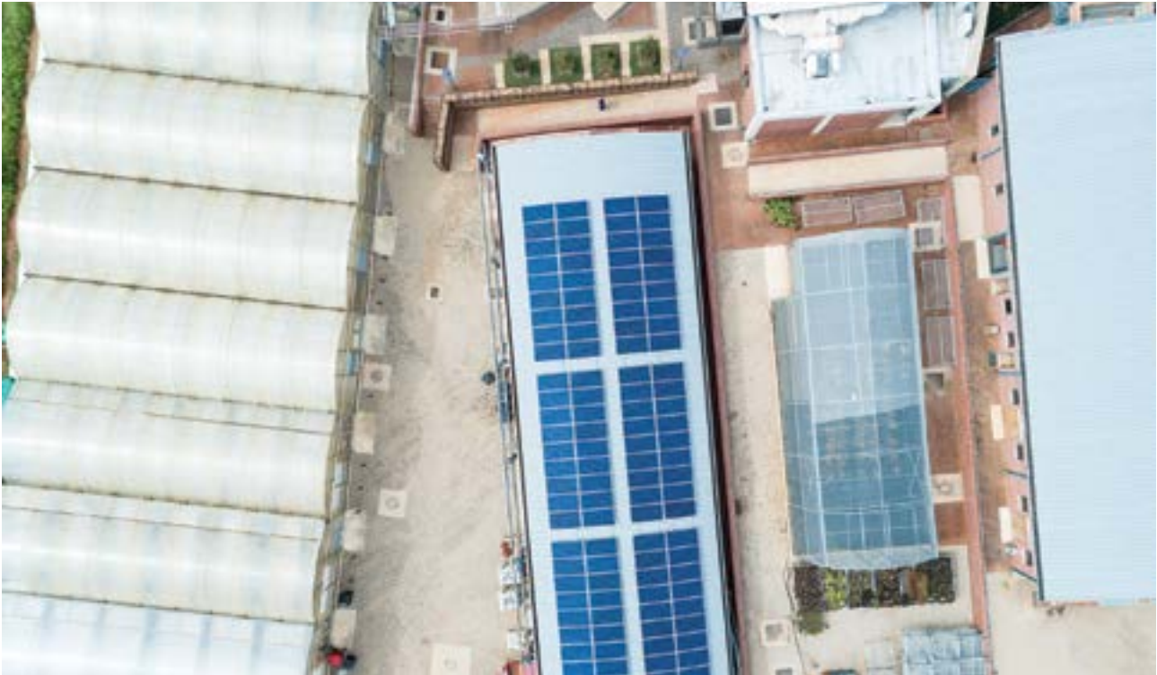
The Horticulture Centre at the science campus was fitted with solar panels to supplement the energy supply, and these came onstream in August 2018. The 35 kilowatt peak (kWp) rooftop solar panels enable the greenhouse to function purely on energy harvested from the sun via solar panels during daytime. This installation won the Higher Education Facilities Management Association (HEFMA) renewable energy award in October 2018.
