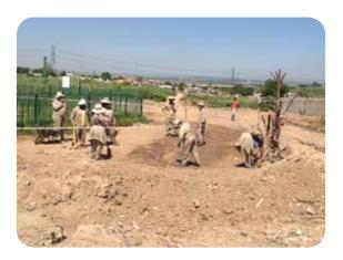
Figure 14: Community workers levelling the swale profile before planting.
