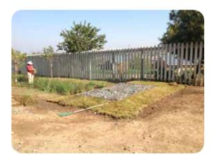
Figure 19: Grass planting around the reno mattress and sedimentation for erosion protection.
