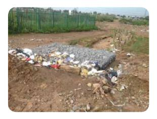
Figure 16: Reno mattress placement on top of sedimentation tank completed; soil levels still need to be completed.
