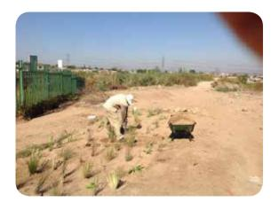
Figure 18: One of the community workers employed for the post completion maintenance clearing the swale from sedimentation after a rain event.
